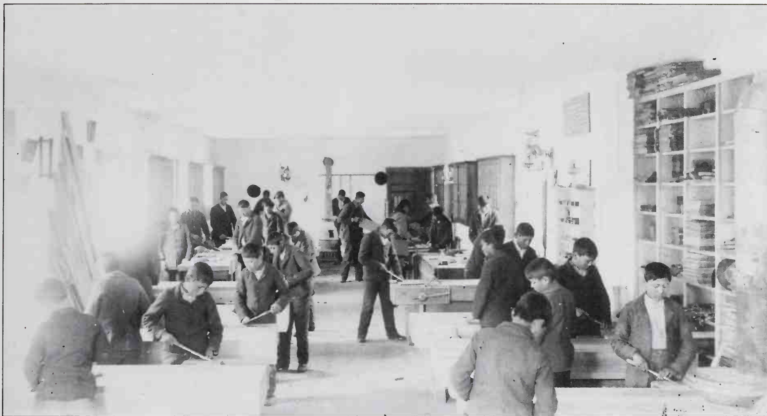
4.37 ABOVE Indian boys in a school carpentry shop. By an unidentified photographer.
