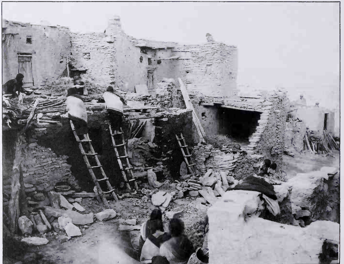
6.15 RIGHT Hopi women building adobe houses in one of the first photographs ever taken of Oraibi Pueblo, Arizona. Taken, despite 'the unfriendly attitude of the natives', by John K. Hillers or the Mindeleff brothers on December 19, 1882.
